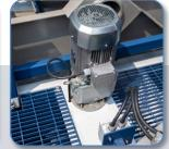
Three 5HP top-mounted agitators with gear-boxes are coupled with a series of mixing guns.
