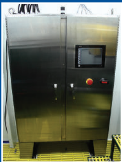
Cabinet Enclosure with Integrated Touch Screen Human Machine Interface (HMI)
